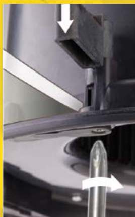
Tighten screws so clips clamp onto ceiling board.
